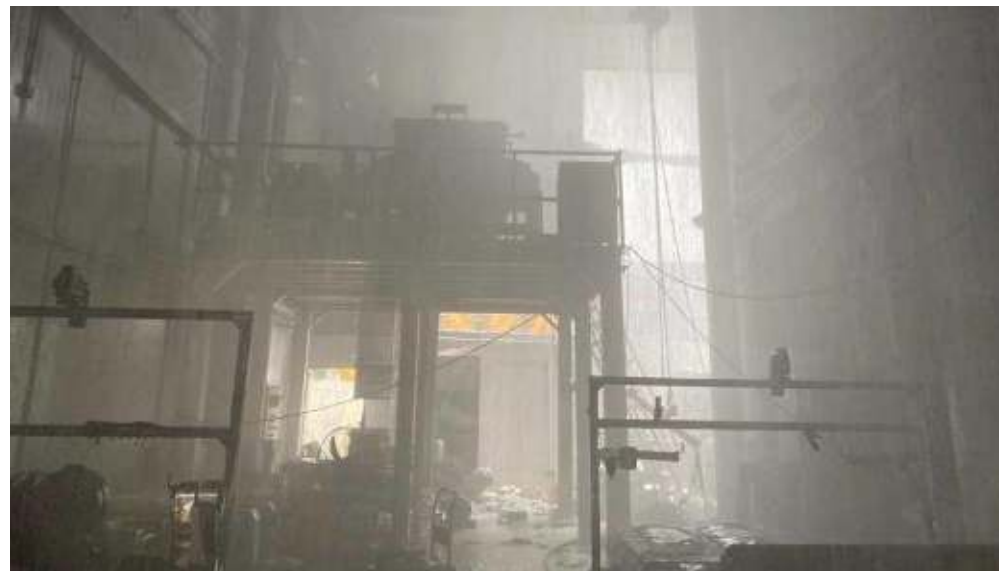
Smoke-logged building after explosion in Tuas, Singapore Source: Facebook/SCDF
